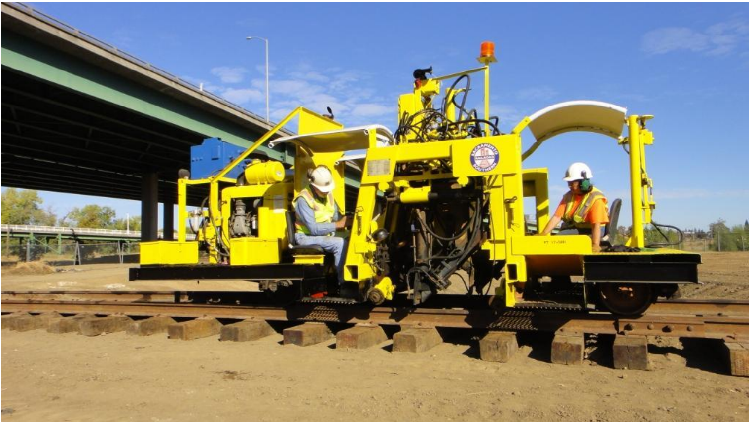
Bring in the Super "B"! Alan and Mike H. operate the spiking guns as Pam loads spikes
