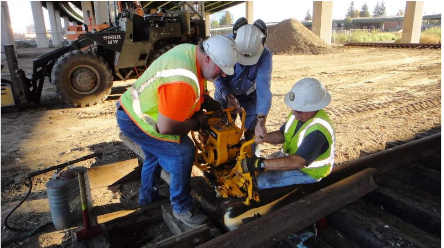
Frank, Alan, and Mike H. attach the rail-drill to the rail-head of one of the panel-track rails
