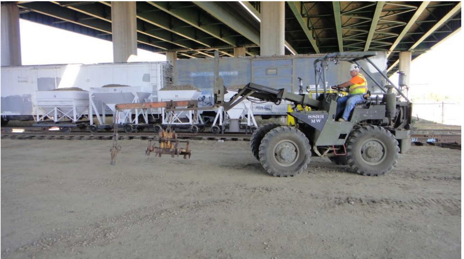
Now it's time to get the track-panels into place. Mike F. brings in Big Green with the stinger, rail tongs, and panel-track lifter attachments
