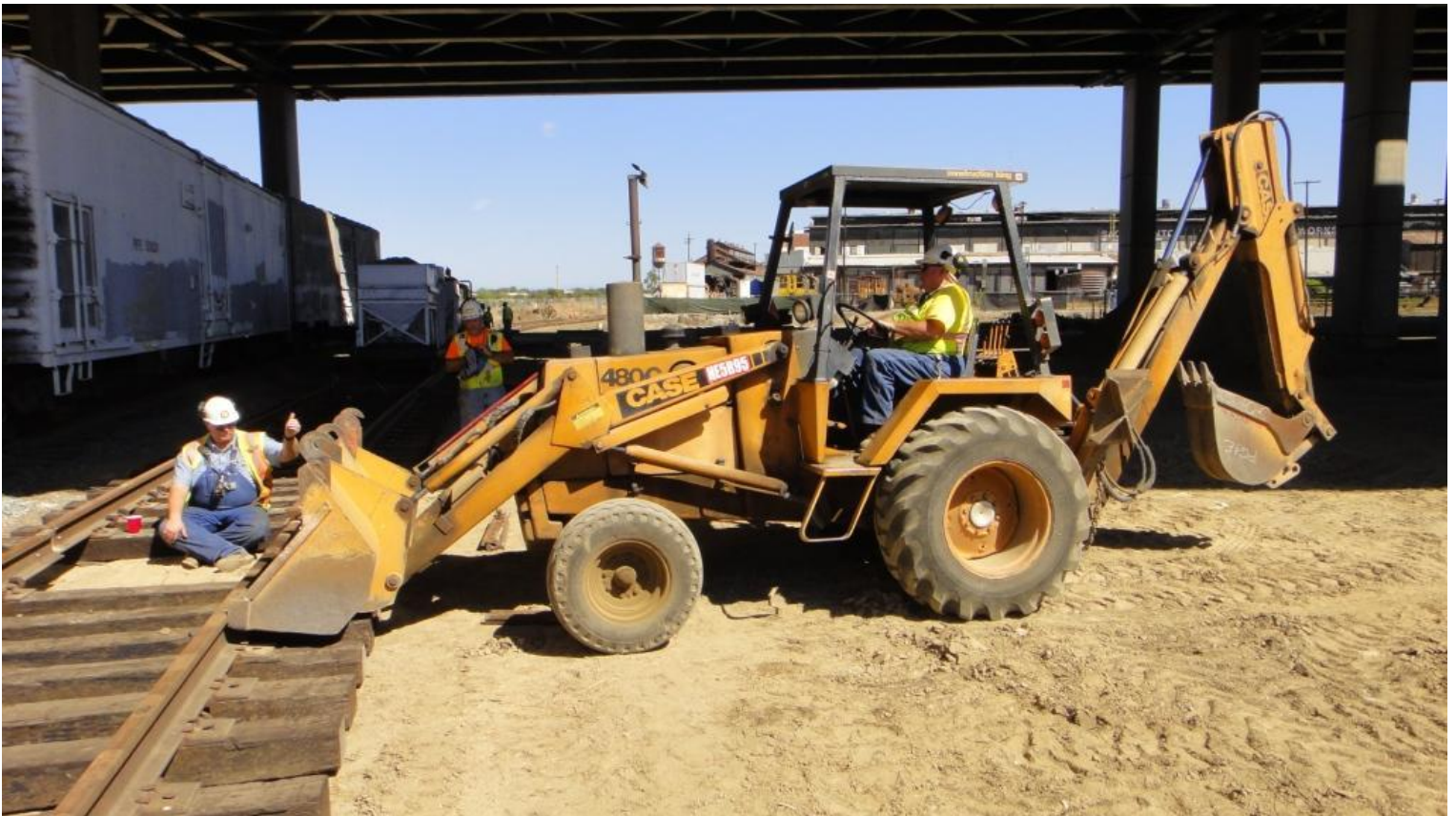
Chris signals, "thumbs-up" to Harry on the back-how as he gives the track a little shove into perfect alignment
