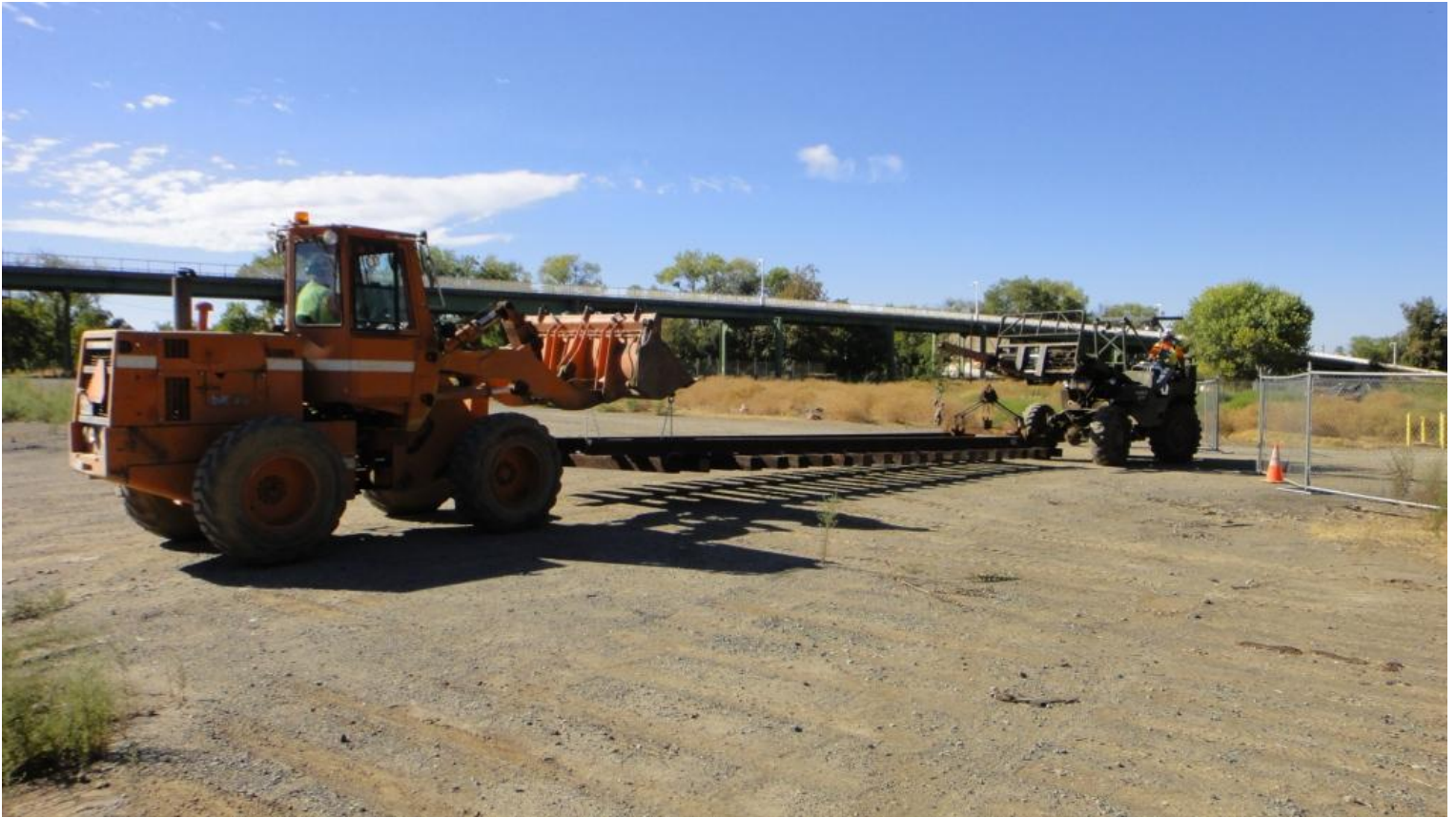
Frank in the loader and Mike F. on Big Green move yet another segment of panel-track to the job-site
