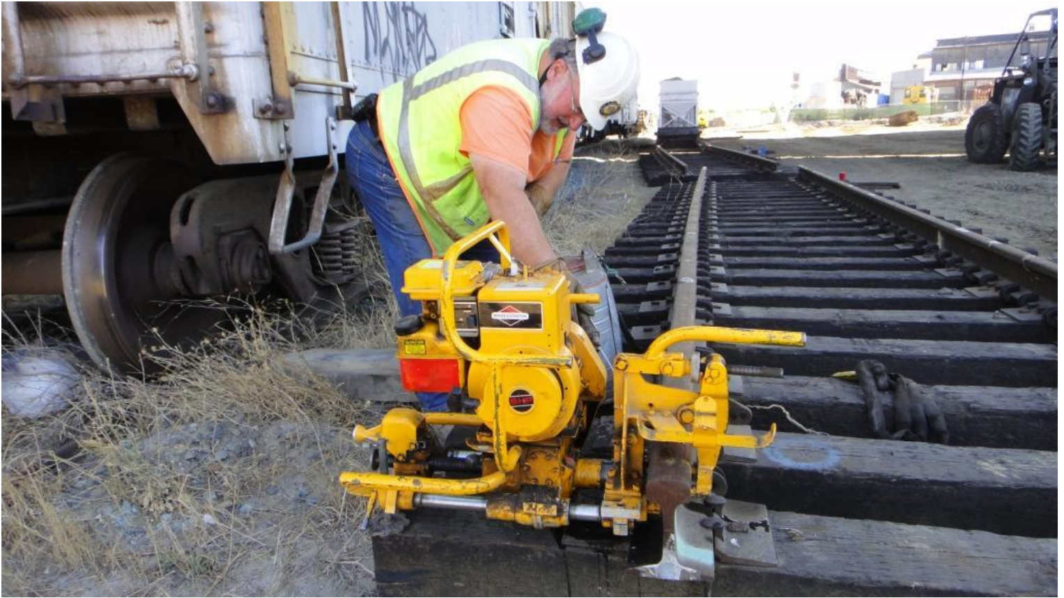
Frank shoots a stream of water onto the drill-bit to keep it cool as it cuts through the web of the rail
