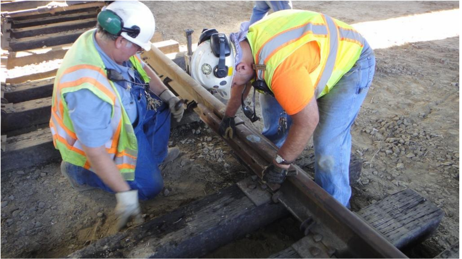
Chris and Mike F. install joint-bars
