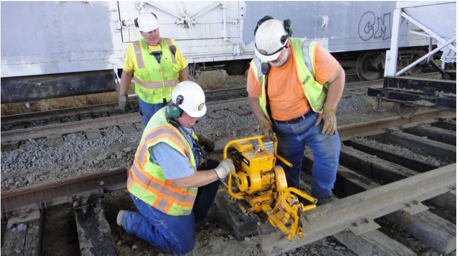
Harry, Chris, and Frank line the rail-drill to the proper position for drilling a bolt hole
