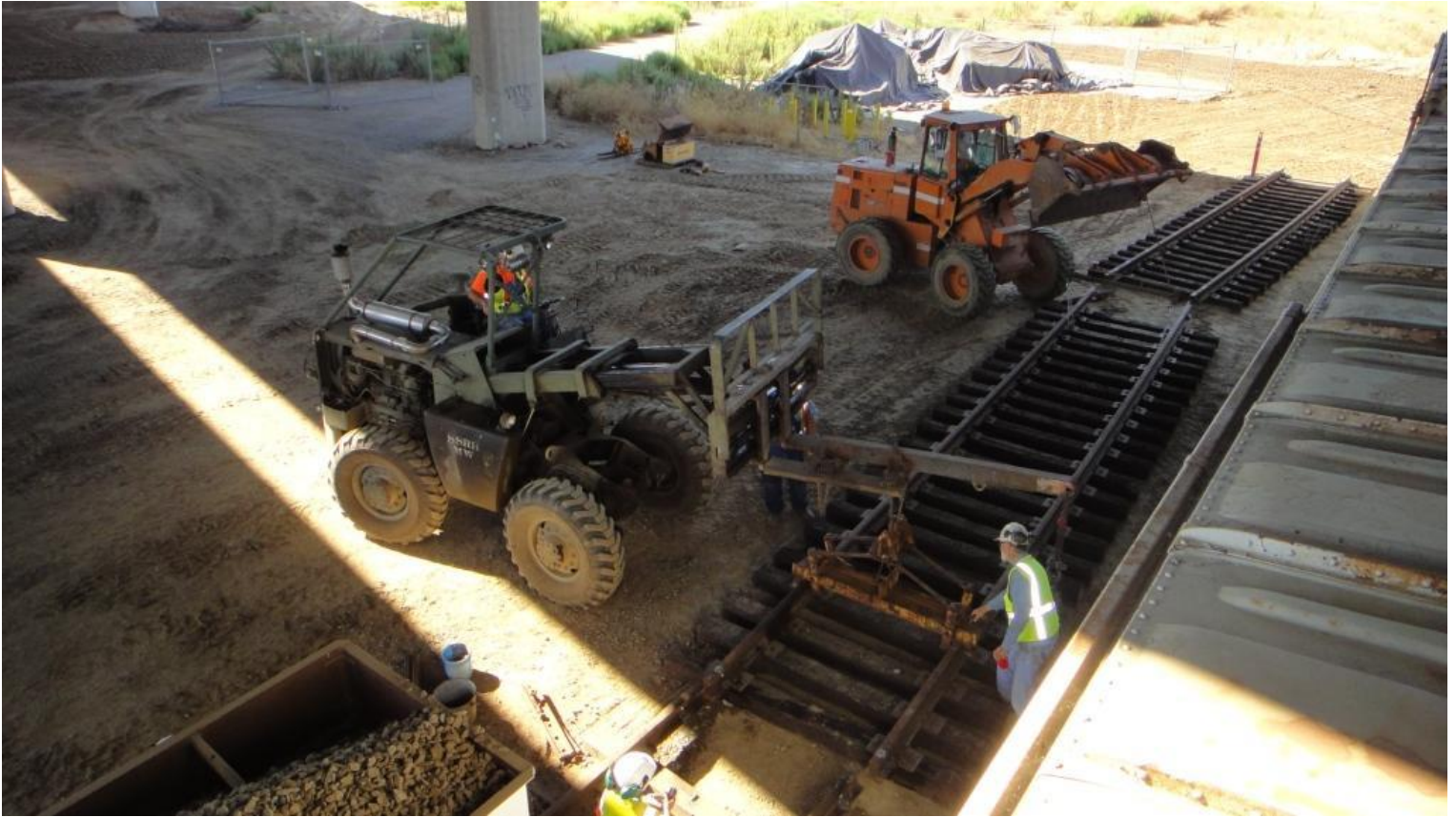
Alan guides Mike F. on Big Green and Frank in the front-end loader in maneuvering the track-panel into the perfect position
