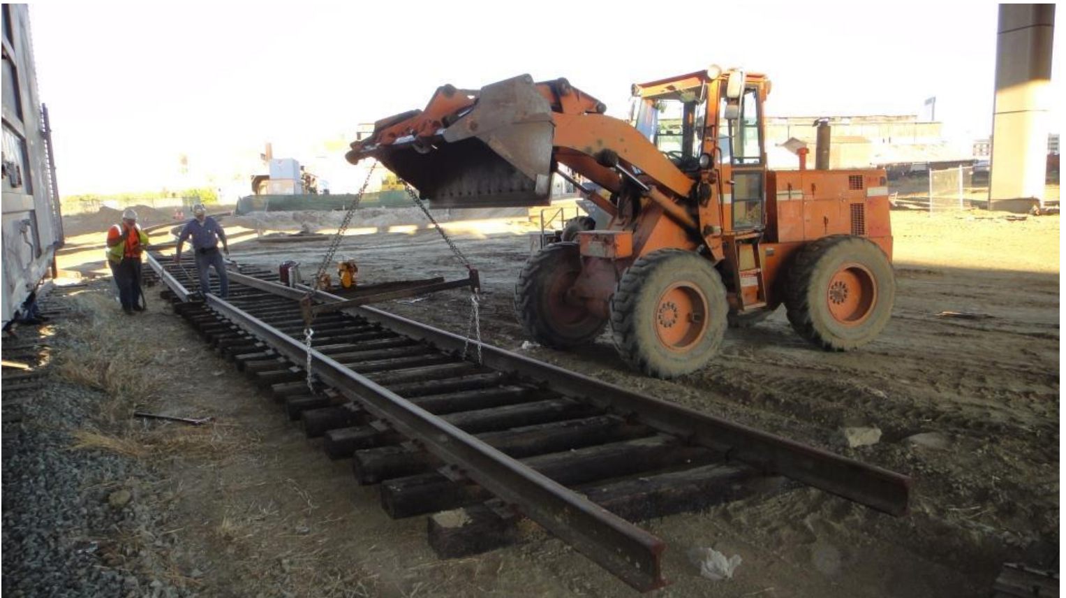
Mike H. in the loader lifts the panel-track section as Frank and Alan guide it into position
