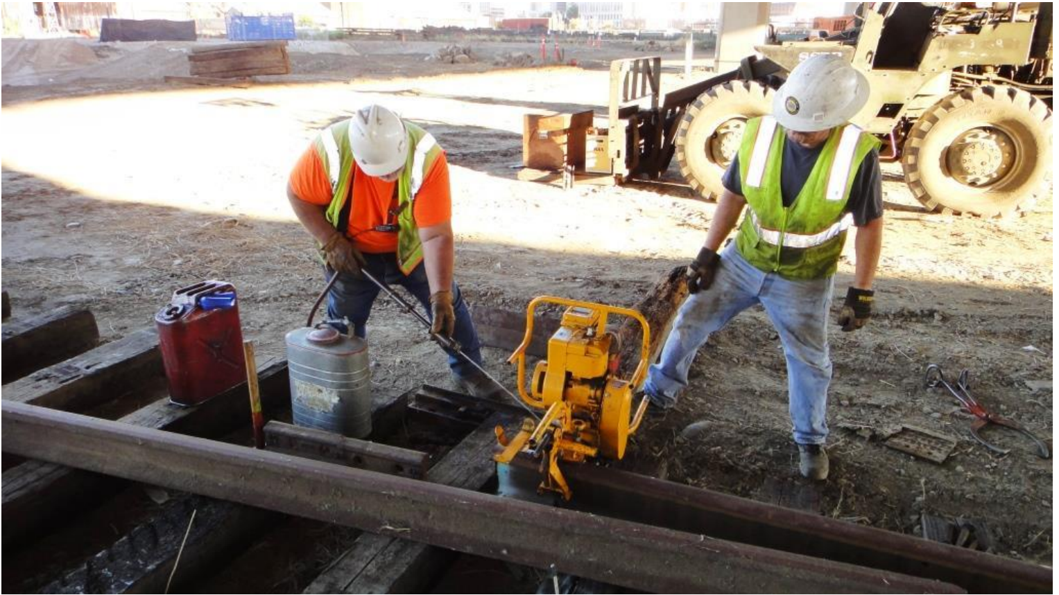
Mike starts-up the rail-drill while Frank sprays water to cool the drill-bit as it cuts through the web of the rail
