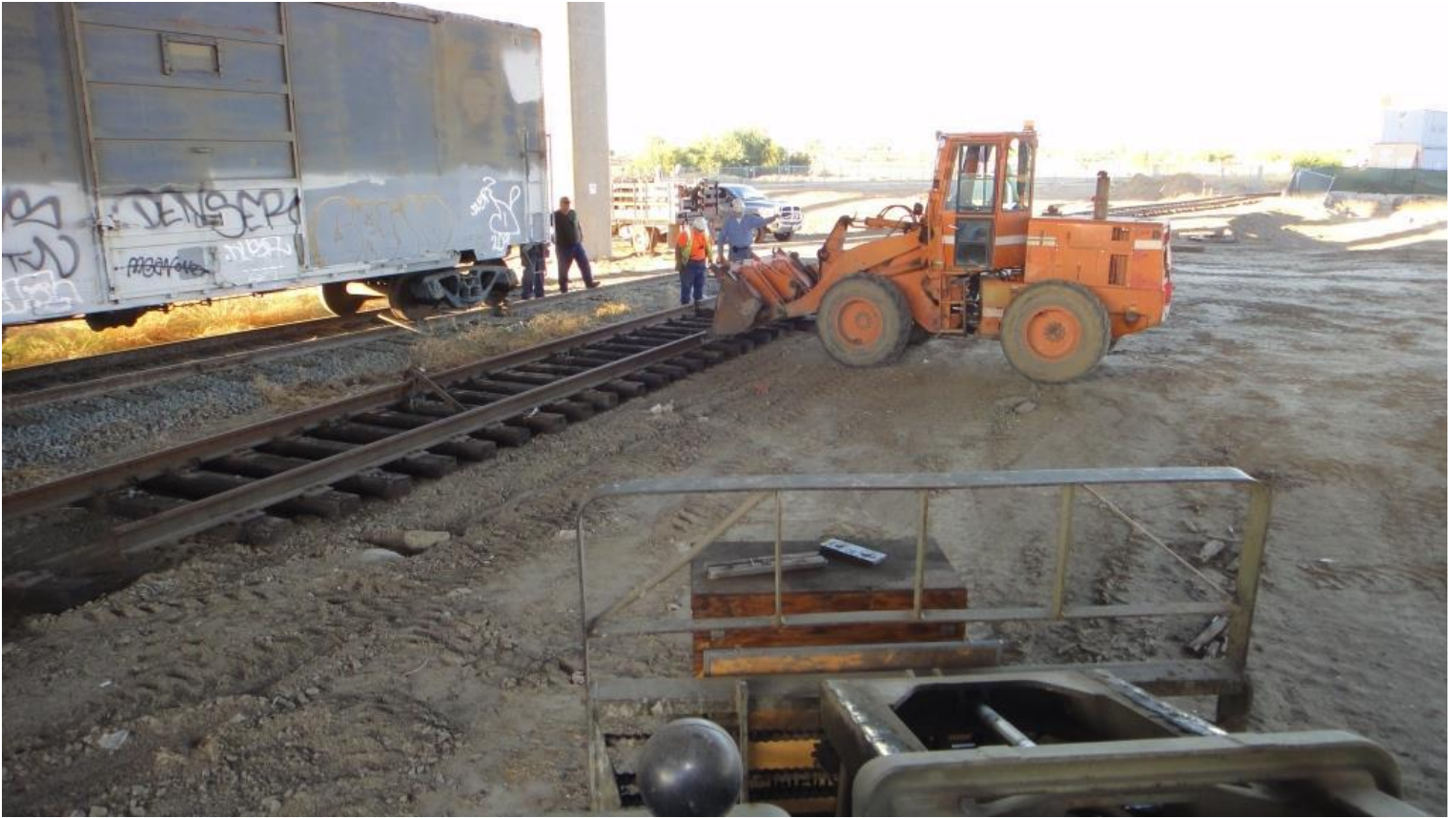
One final push from Mike H. in the loader lines up the rails perfectly
