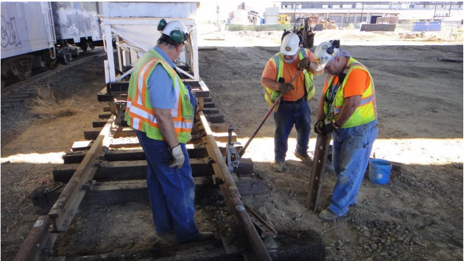
Chris surveys the situation as Frank jacks-up the east rail to line up with the west. Mike F. brings in a joint-bar
