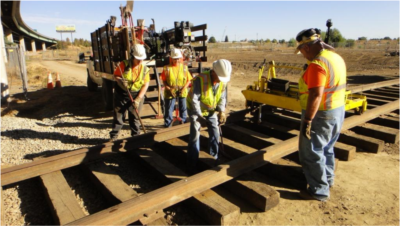
With the rail-lifter lifting the rails, Mike T., Heather, and Pam square-up a tie as Mike F. looks on
